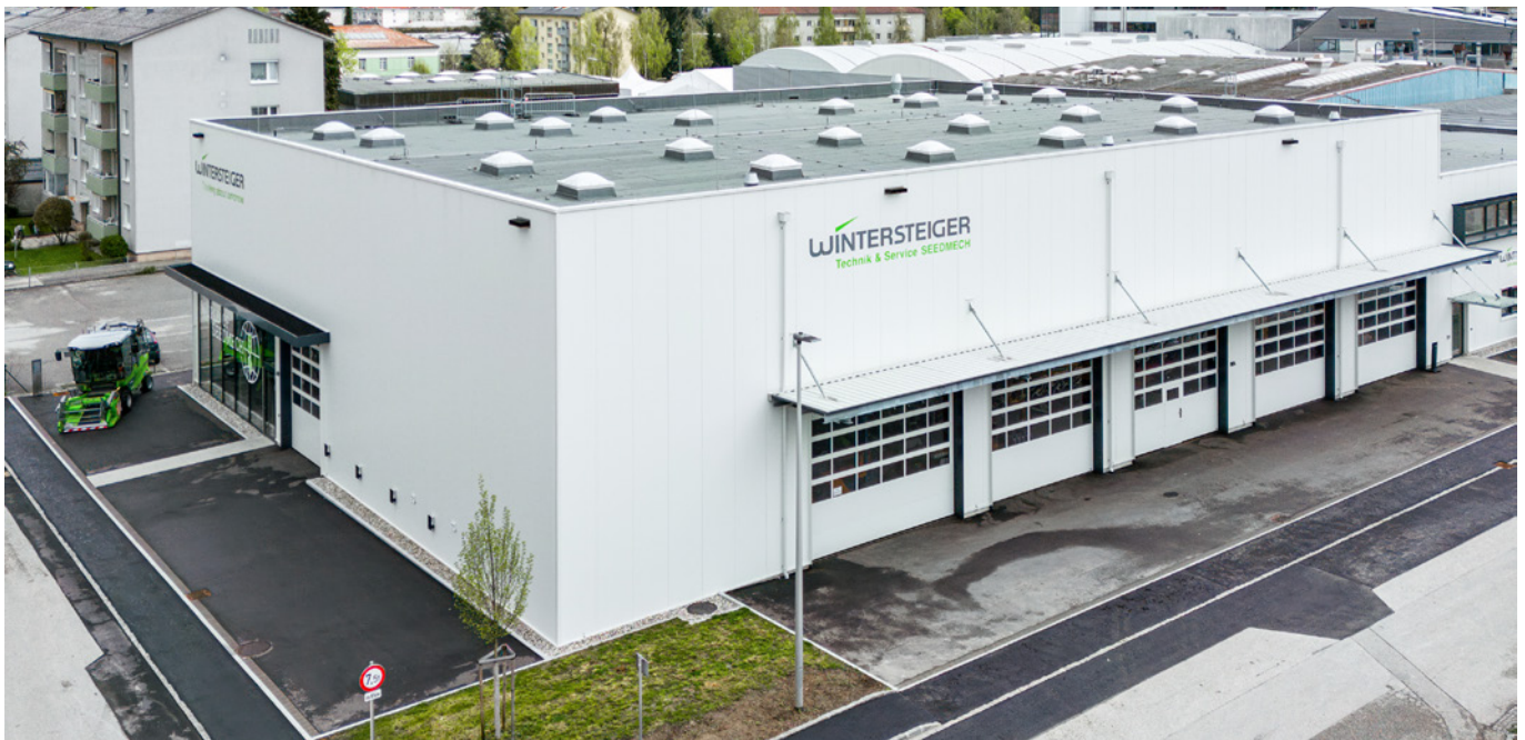
New building 2022: Technology & Service Seedmech
